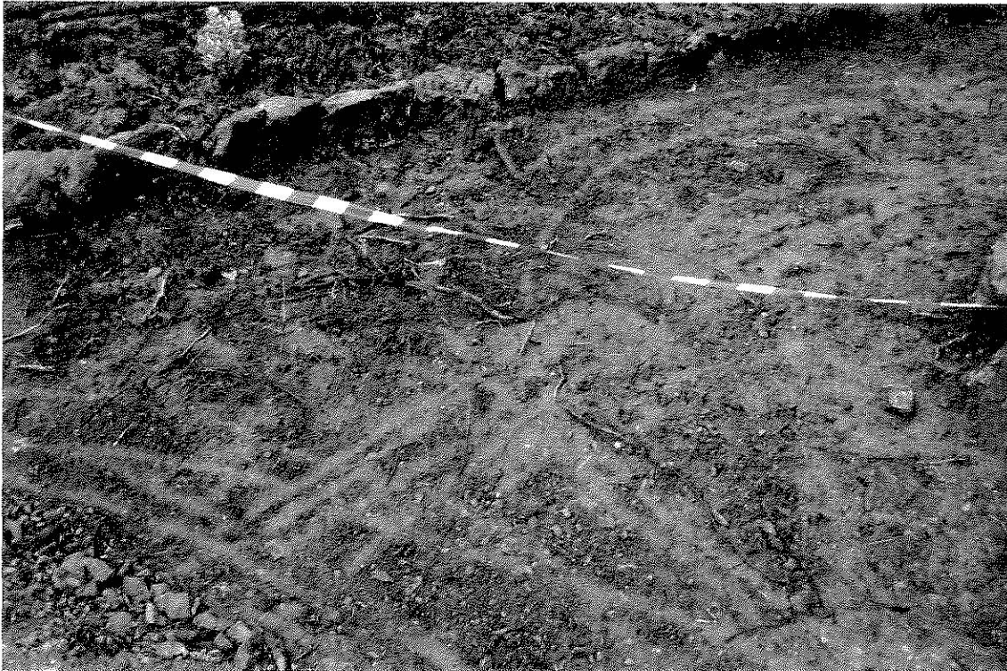
Exposed damaged roots - recent development works to front of church.
